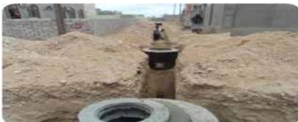
sanitation network project –Alghaida City.
