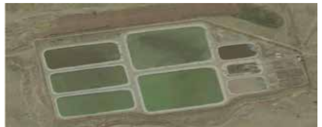
Wastewater treatment plant -Beit AL-Faqeeh city.
