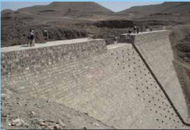
AMLAH ALMALHA WATER BARRIER--STORING CAPACITY : 82023 M3
