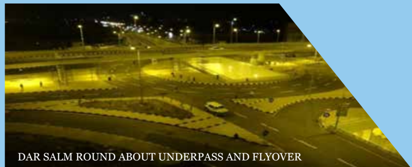
DAR SALM ROUND ABOUT UNDERPASS AND FLYOVER -SANA'A
