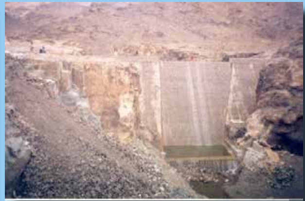
BENI QAWS WATER BARRIER STORING CAPACITY: 45260 M3
