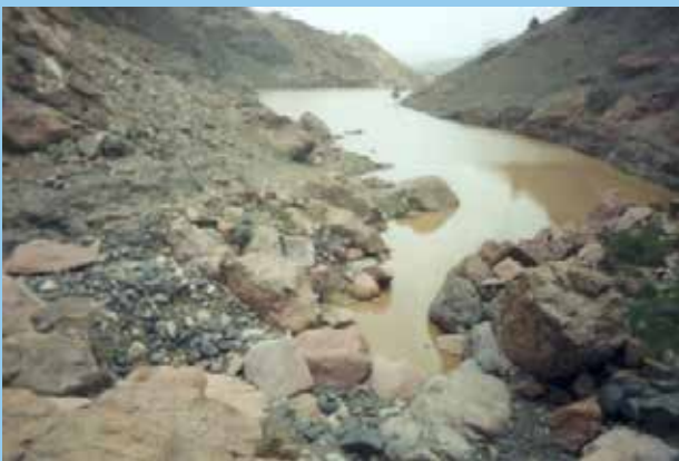
260000 BENI QAIS DAM-STORING CAPACITY :260000 M3
